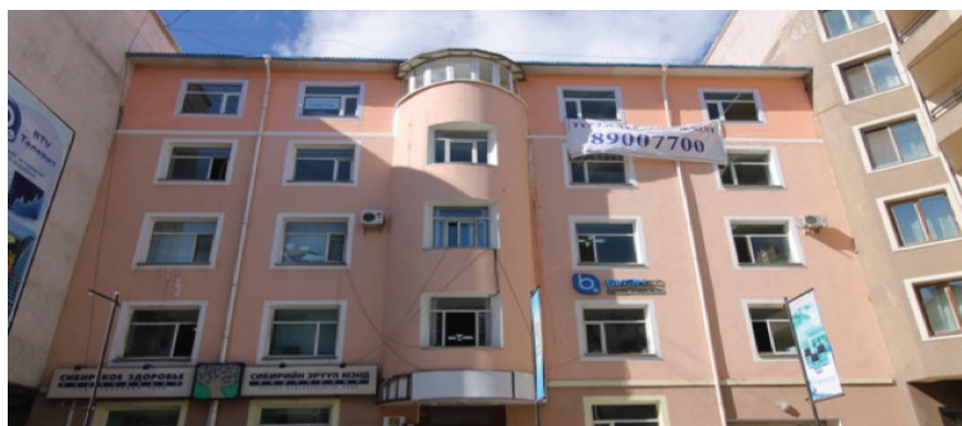
Before renovation of Denver Exterior
