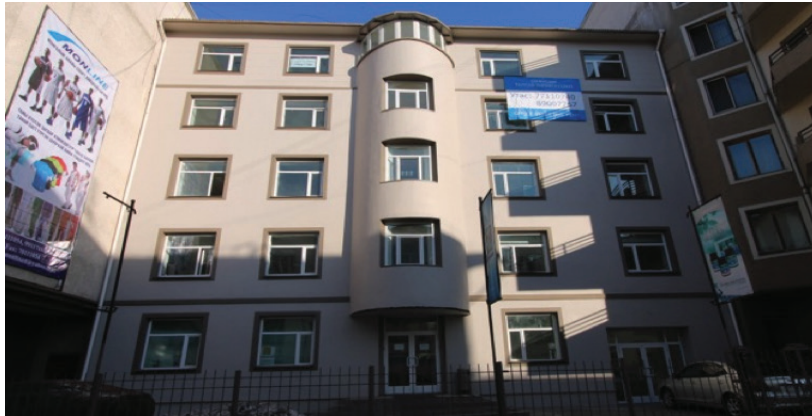
After Renovation of Denver Exterior
